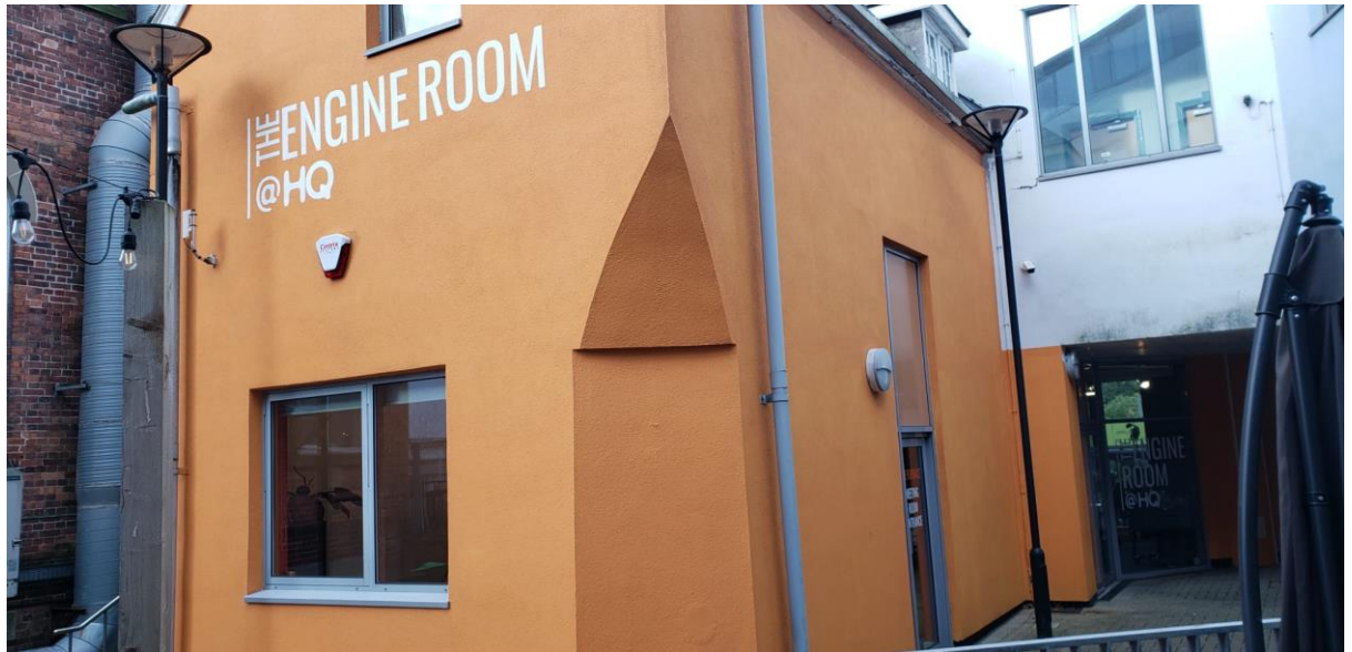
Figure 14: HQ Swansea, collaborative CCI led workspace.
